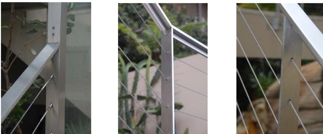
Figure 4. Balustrades cleaned using the Electropolsih process.
